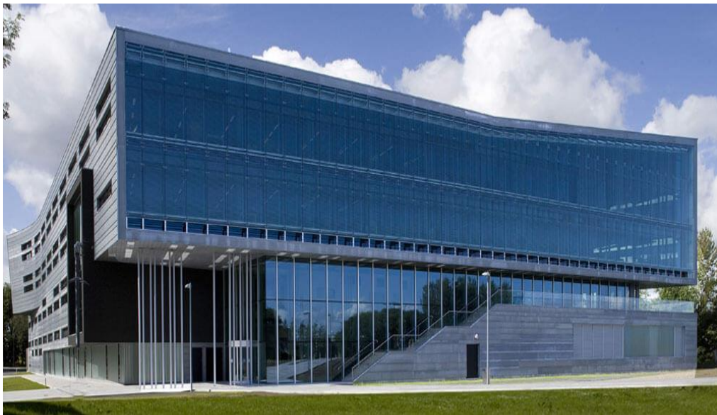
Figure 4.2: Alice Perry Engineering Building at the National University of Ireland, Galway (NUI Galway).
