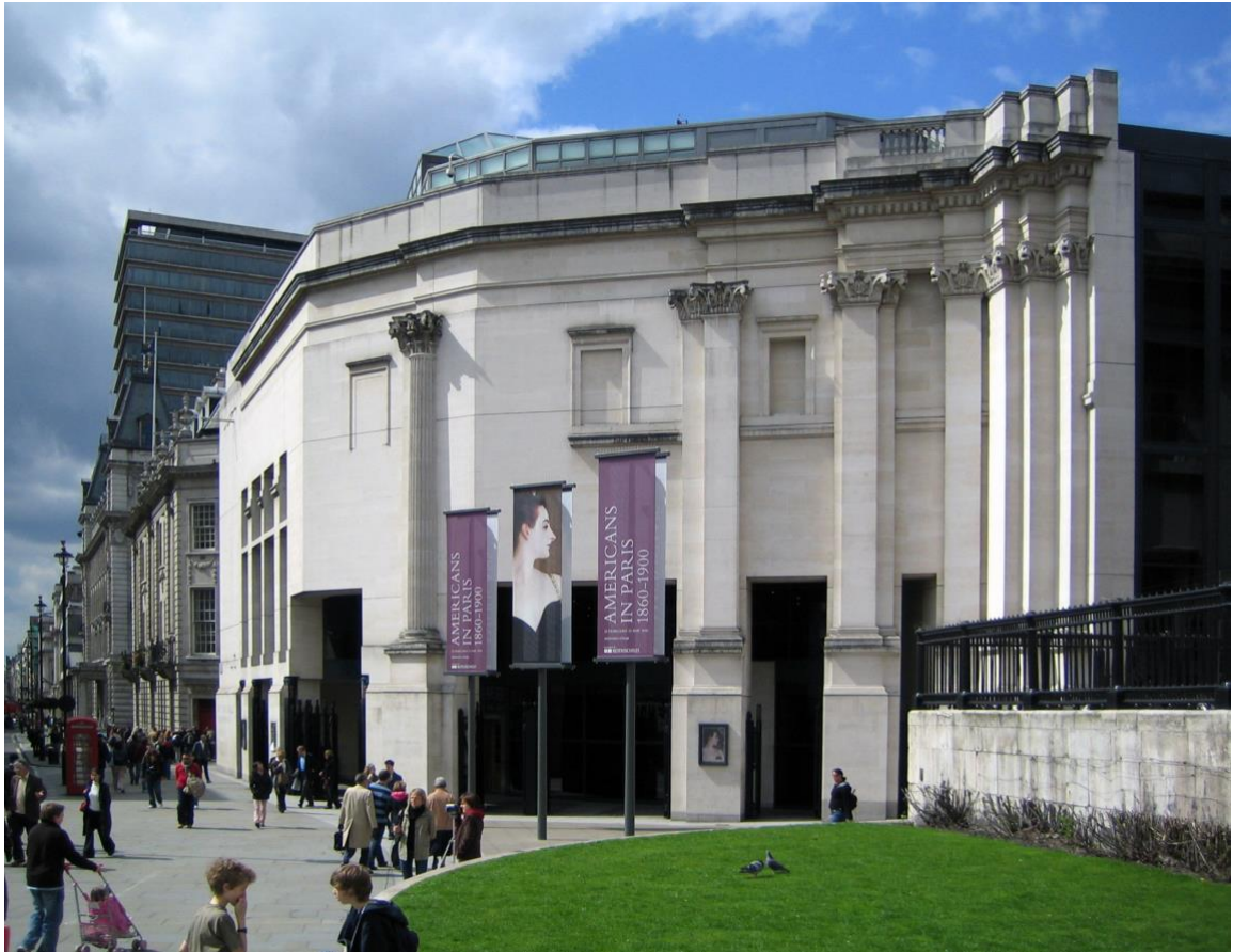
Figure 22 National Gallery Extension, London UK, 1989-1991 (Architects Robert Venturi, Denise Scott Brown and Associates Photograph by Richard George - Own work, CC BY 2.5, https://commons.wikimedia.org/w/index.php?curid=715349 )
