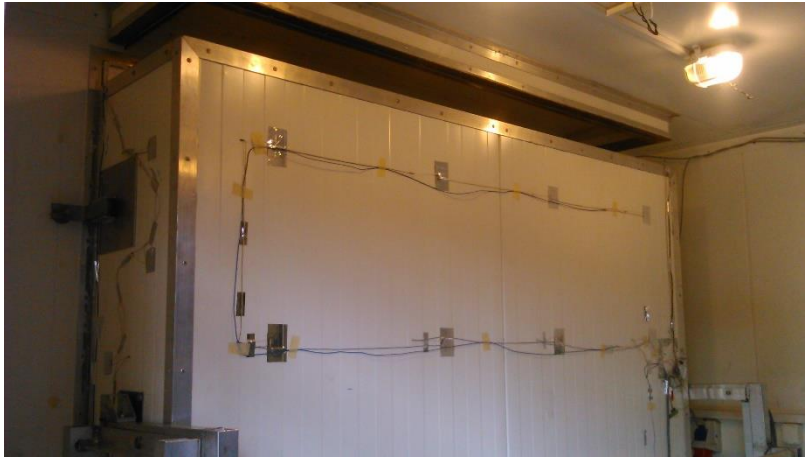
Fig. 3. Metering box fastened to the surround panel.
