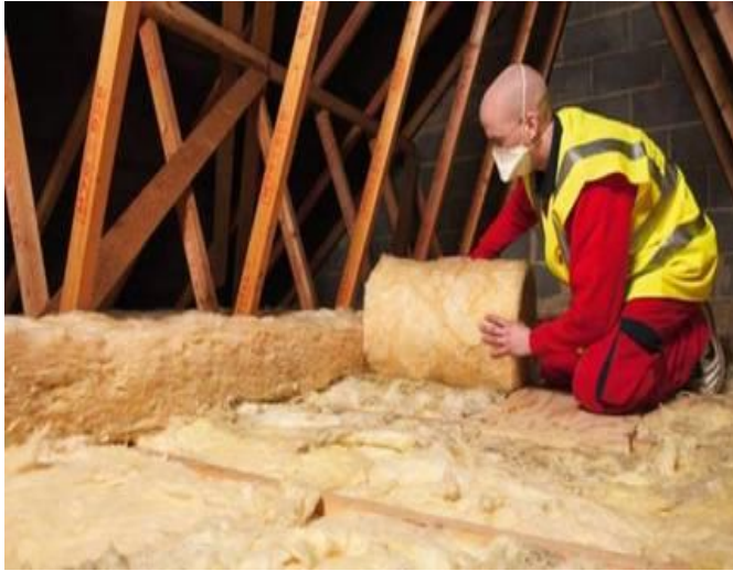
300 mm thick mineral wool insulation
