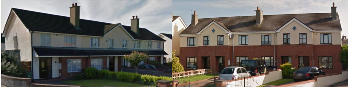
Figure 2(a) Mid- and end-terraced houses constructed in 1994 and Figure 2(b) Mid- and end-terraced houses constructed in 2000
