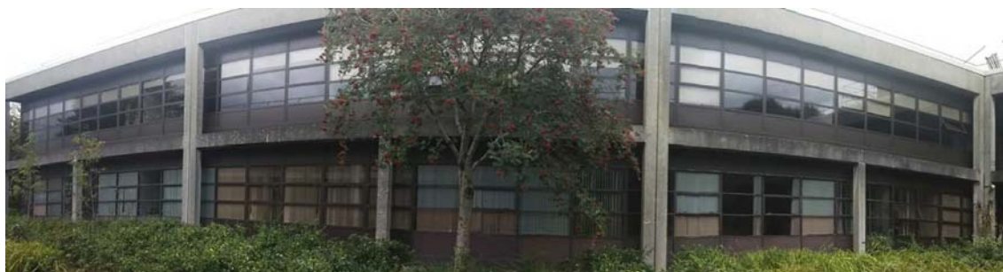
Figure 3 Panoramic view of the building
