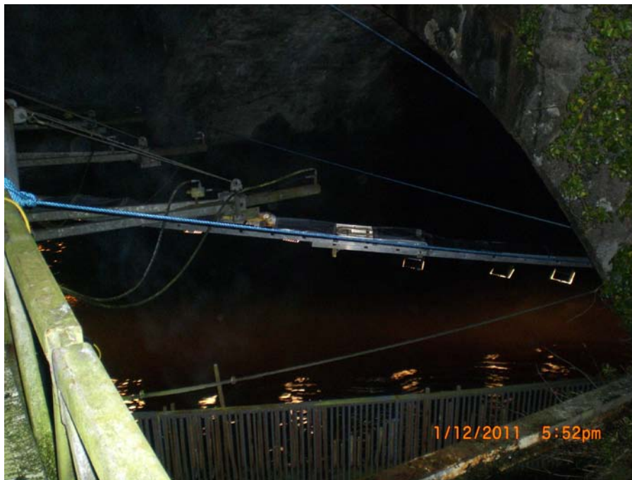
Fig 5.1 Photo of the light barrier at arch 5 of Killaloe eel weir.
