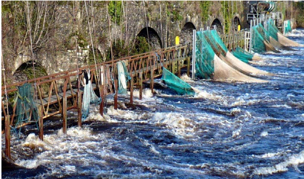
Fig. 1.6 Killaloe eel weir, viewed from downstream. Note that the nets are not set in this photograph.
